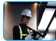
■ Adjusting the camera angle at the elevator
